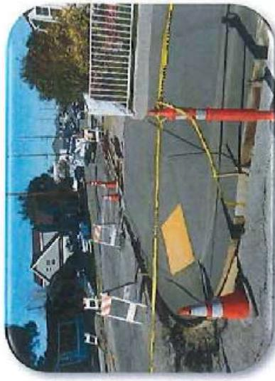
Project Description: This project will construct new curb ramps in conformance with State and American with Disability Act guidelines and replace damaged sidewalks.
