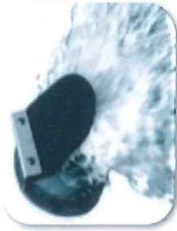
**Project Description:** This project will replace the East Antioch Creek outfall near the intersection of Fulton Shipyard Road and McElhaney Road. The work will include replacement of two sections of storm drainpipe with associated flapper gates and reconstructing a deteriorating sanitary sewer pipeline that crosses the outfall piping.
