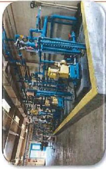
Project Description: This project will install flow paced pump meters and motors for chemical introduction at the Water Treatment Plant.
