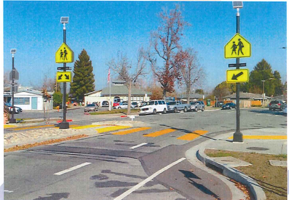
Rectangular Rapid Flashing Beacons (RRFB)
