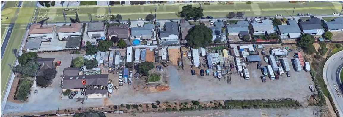
Site 124 (+701 Wilbur Avenue)
