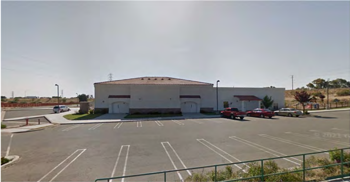
Site 164 | 3415 Oakley Road
