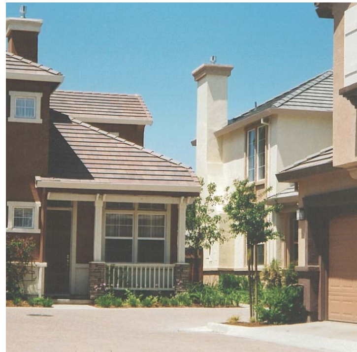
Well Articulated Elevations in a Private Lane Neighborhood
